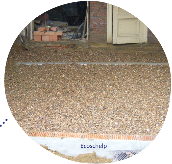
Schells as dry screed insulation
